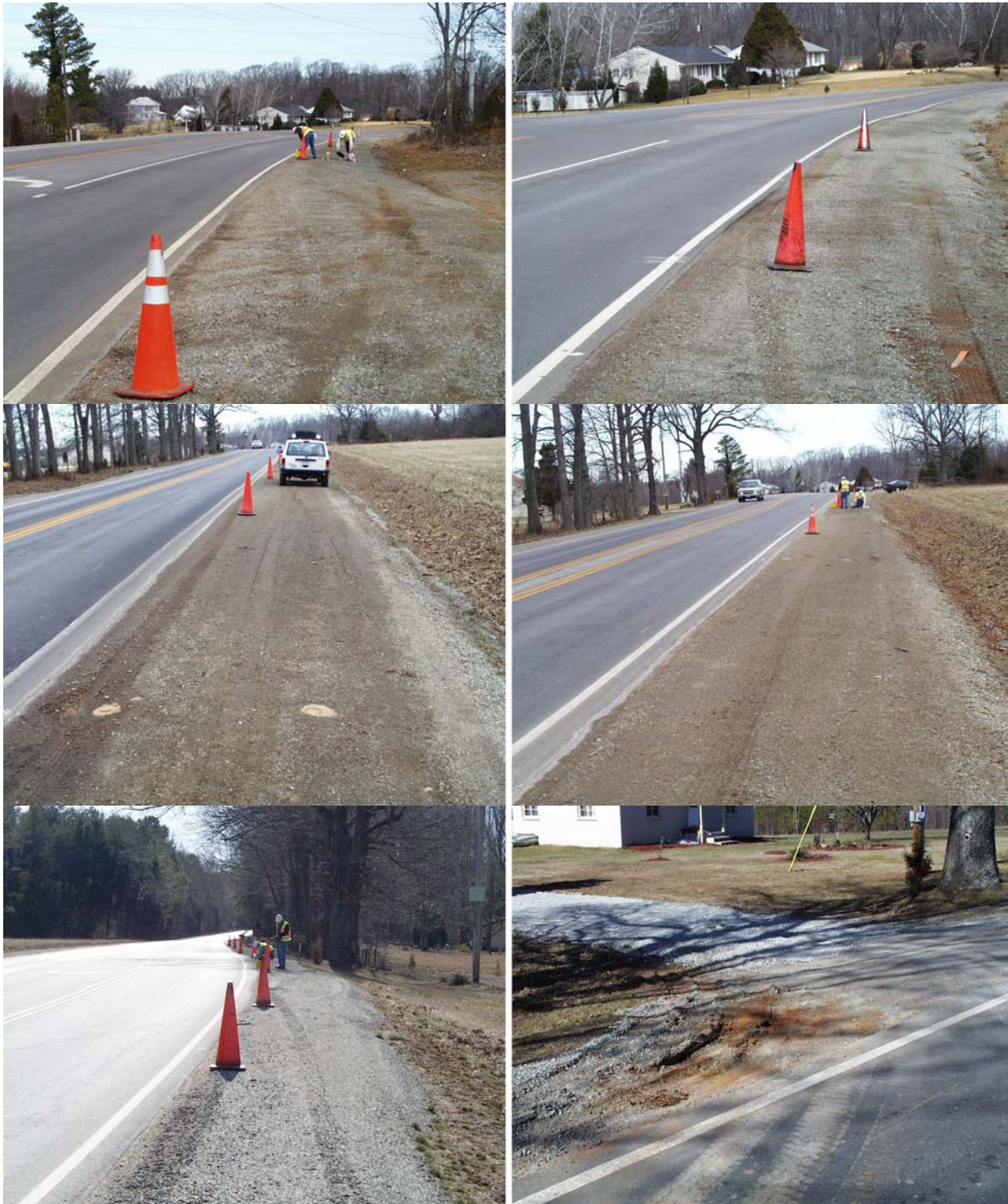
Figure 5. Test and Control Sections, 2/8/2005. Top, Soiltac; middle, Centrophase AD; bottom, control.
