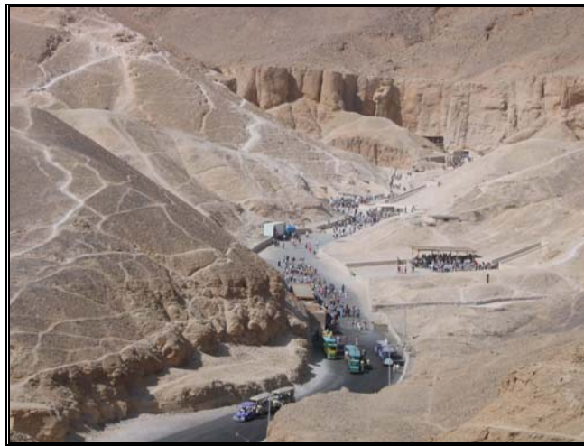
Figure 74: Existing Road Surface
