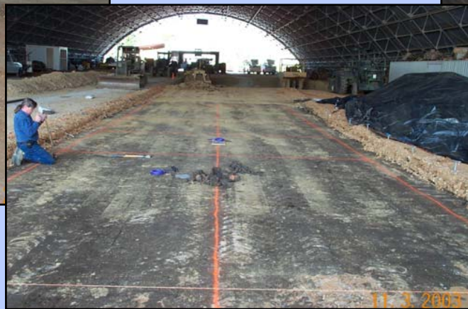
Installing pressure cells at top of clay subgrade
