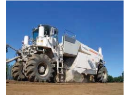
Road Base & Sub-Base Road Base Stabilization Sub-Base Stabilization Mud Suppression
