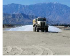
Land Development Fugitive Dust Control Erosion Control Silt Loading Control
